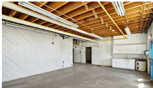
Building 1 - Multi-purpose/Break Room
