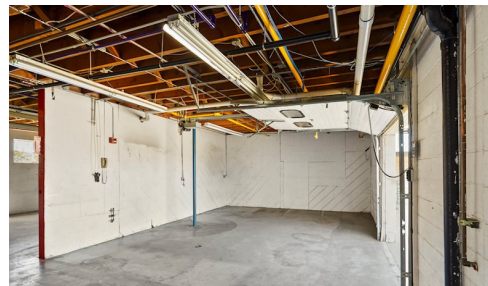
Building 1 - Receiving Dock
